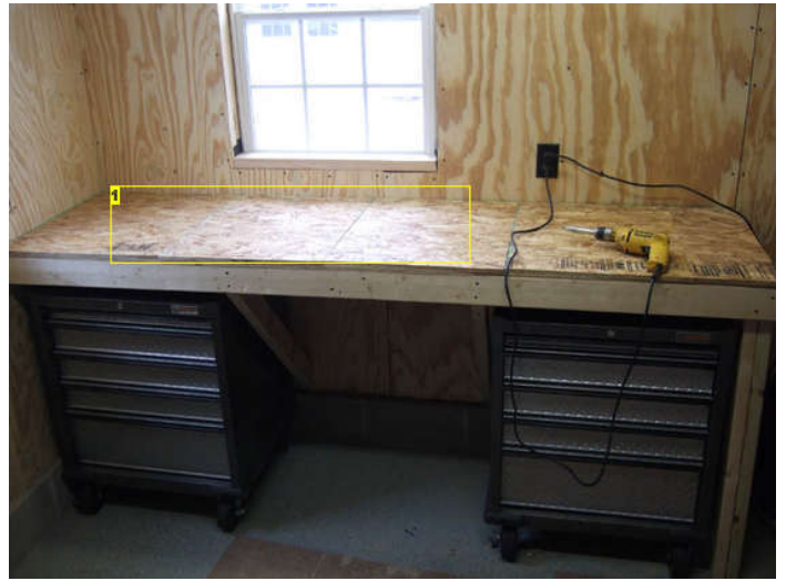
Image Notes 1. final OSB layer. notice there are seams in the top since I didn't have any single pieces big enough. this is no problem.
