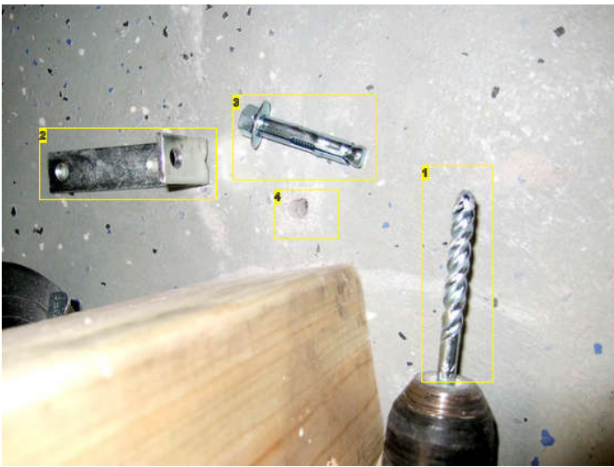
Image Notes 1. masonry drill bit 2. angle bracket 3. 3/8 inch wedge style concrete anchor 4. hole in concrete
