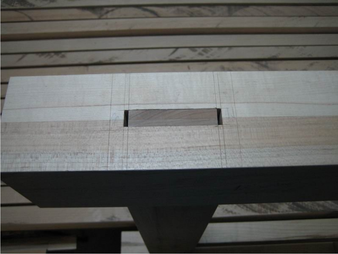
Through tenon showing allowance in mortise for wedges
